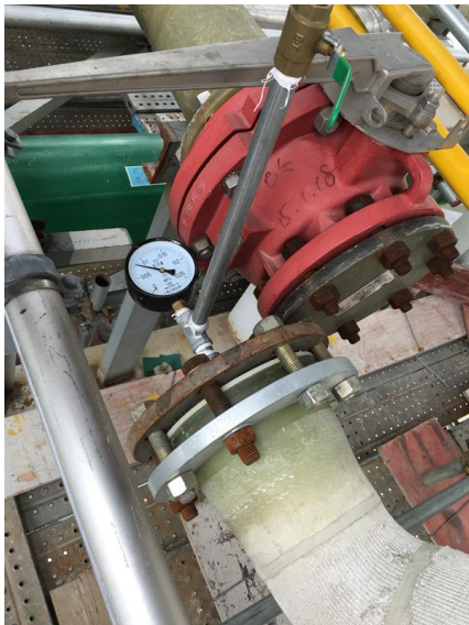
Pressure testing before and after lamination
