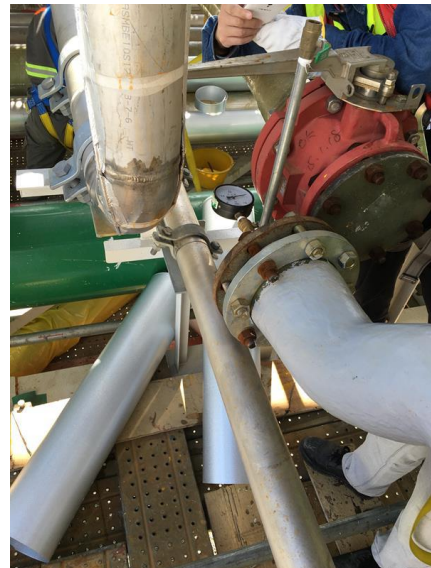
Pressure testing before and after lamination
