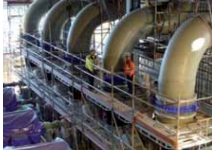
Quality inspection of GRP auxiliary piping on an absorber (D = 1200 mm, P = 10 barg)
