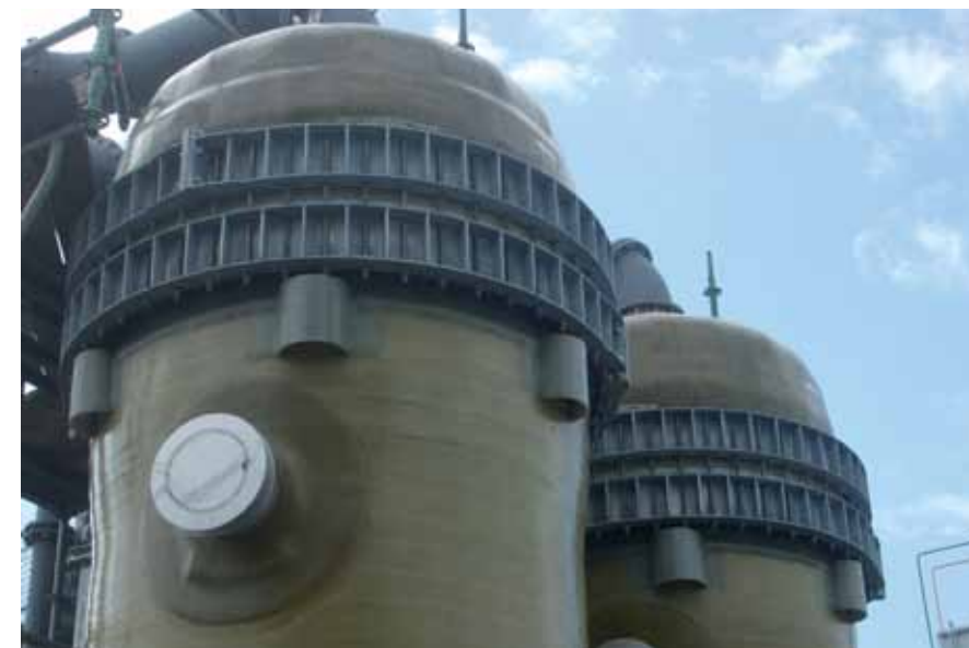
GRP reactors with PED approval (P = 8 barg, T = 80 °C)
