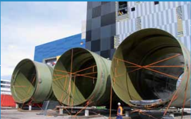
Preparation of a stack liners (D = 8 meter) ready for installation
