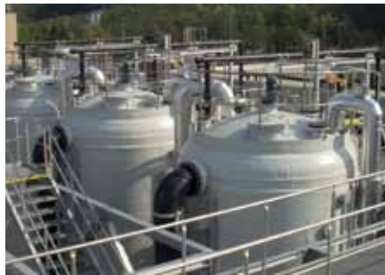
Storage of waste water at 90°C (3 x 120 m³, D = 3500 mm)
