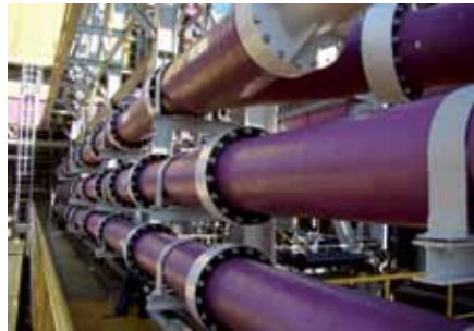
GRP piping, part of the chemical processing at a steel plant
