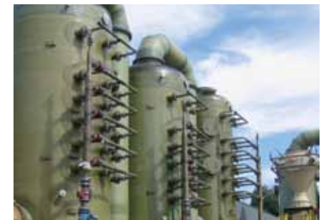
Three GRP scrubber to filter odors
