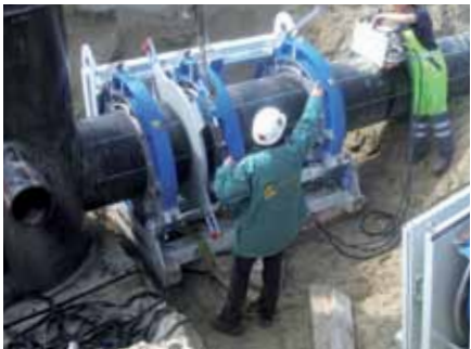
Installation of a thermoplastics (PE) pipe line by butt fusion welding (D = 600 mm)
