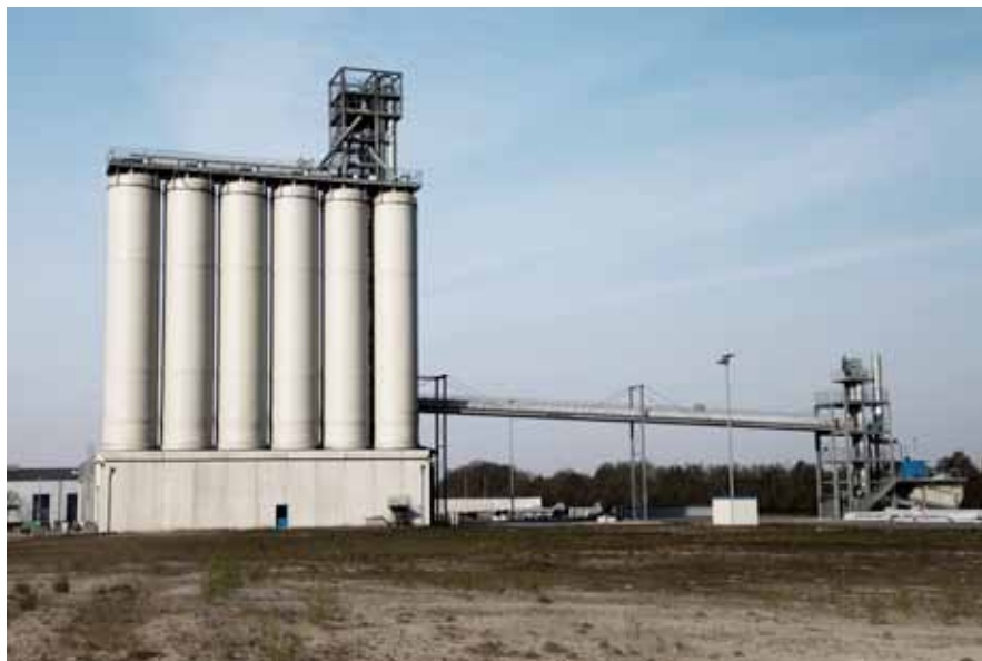
GRP silos (6 x 500 m³, D = 5000 mm)
