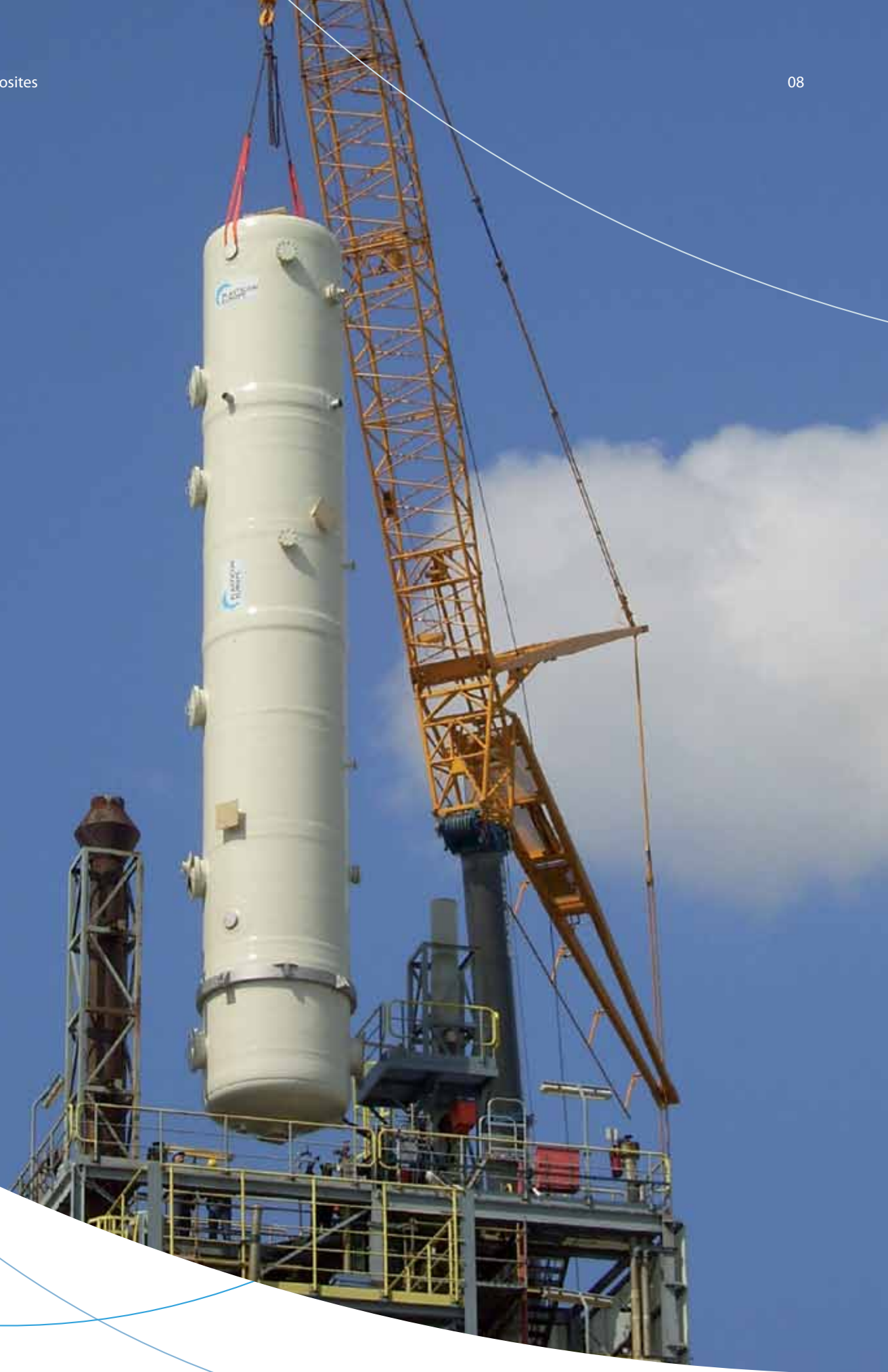
Lifting of a PVDF/GRP column (D = 3.500 mm, H = 16.000 mm)
