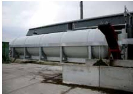
Storage of NaOCl in a specially designed steel construction (100 m³, D = 3000 mm)
